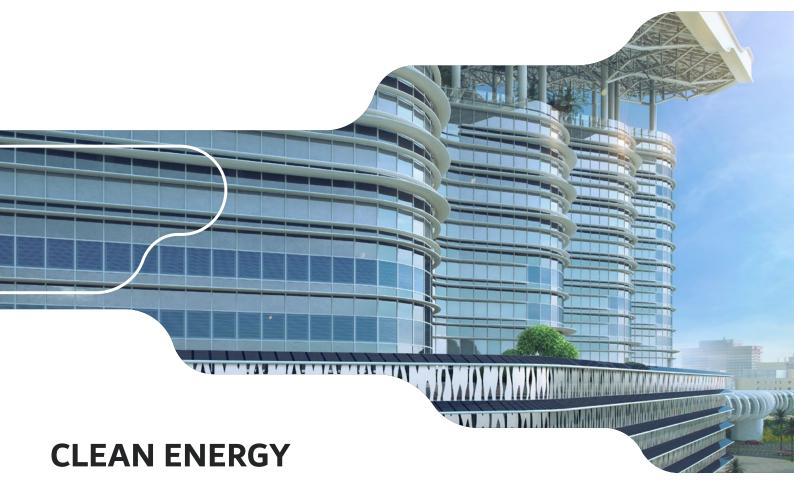
Al-Sheraa's design makes the most of its location to provide the largest possible surface area to generate solar power. The building will generate over 6,500 megawatt hours (MW/h) a year of renewable energy. It will have over 20,000 square metres of photovoltaic solar panels on its roof as well as 1,000 square metres of Building Integrated Photovoltaics.
